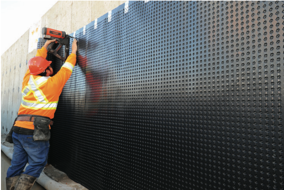
INSTALLING SPEEDCLIPS EVERY 30CM (12")
