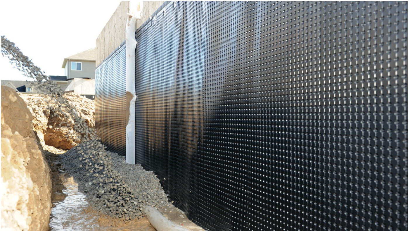
BACKFILLING OVER THE FOOTING DRAIN
