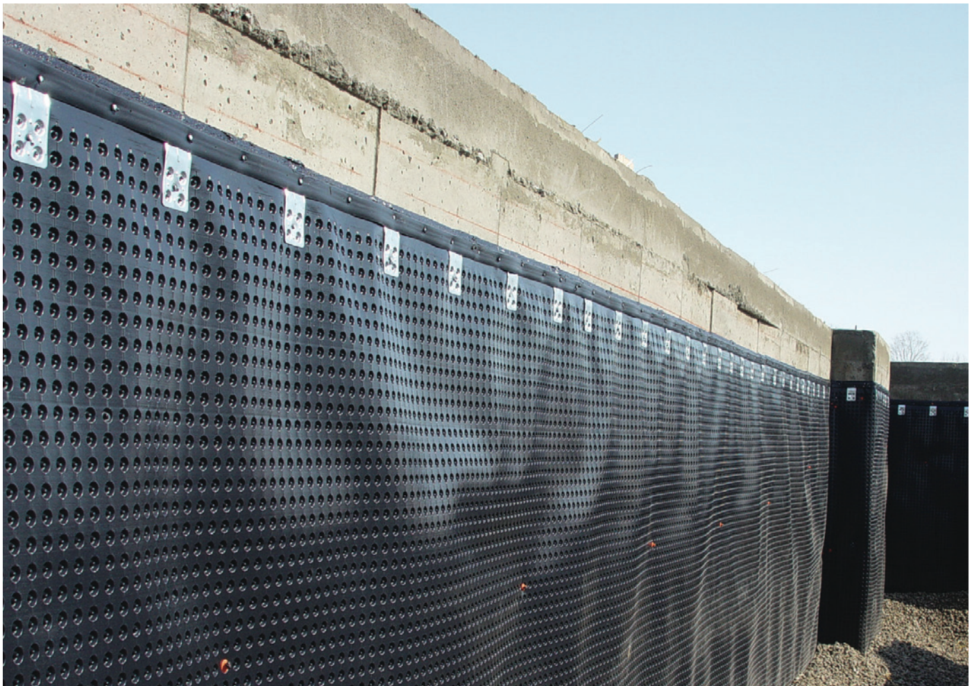
FINISHED INSTALLATION OF PLATON FOUNDATION WRAP
