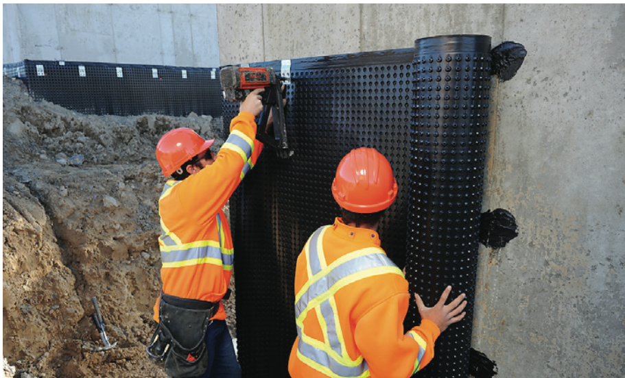
PLATON INSTALLATION - FOUNDATION WALLS
